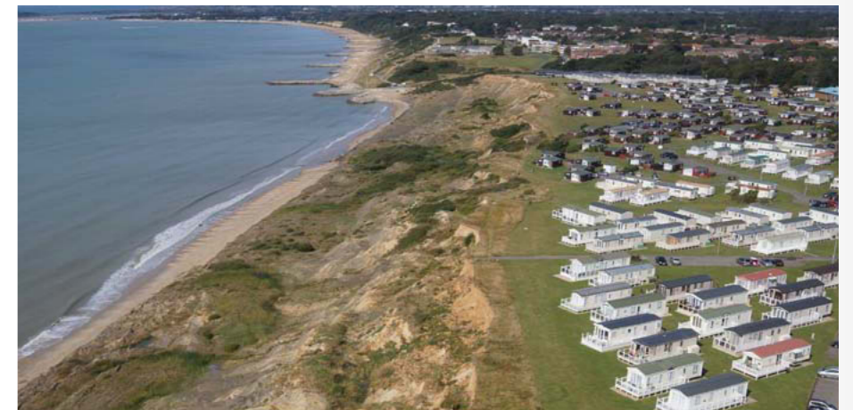
Cause for concern: Properties close to the slip
