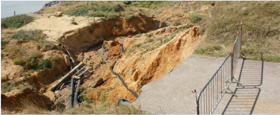
Exposed: Damage caused by the slip
