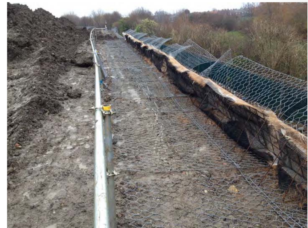
For the redevelopment work at Bell Green in South London, Paradrain and Green Terramesh creates a steep, vegetated-faced wall as part of a reinforced soil, slope construction.
