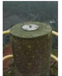
Figure 17 - "Fixed" survey station
