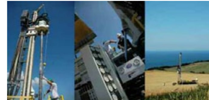
At work: New Sonic rig
