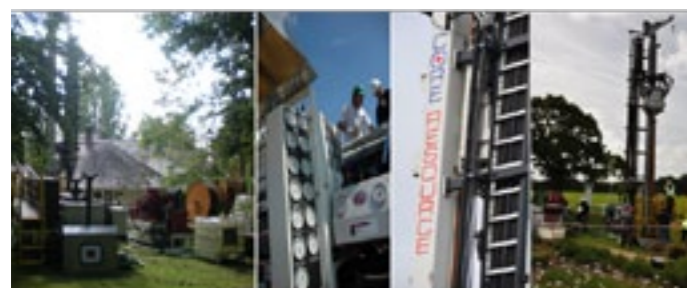
Work on the Isle of Wight
