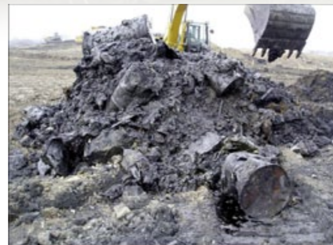
Figure 1: A site declared ready for construction actually contained a large number of discrete buried dumps of steel drums containing waste oil; these were located successfully using magnetometry, excavated safely and cleaned up efficiently.
