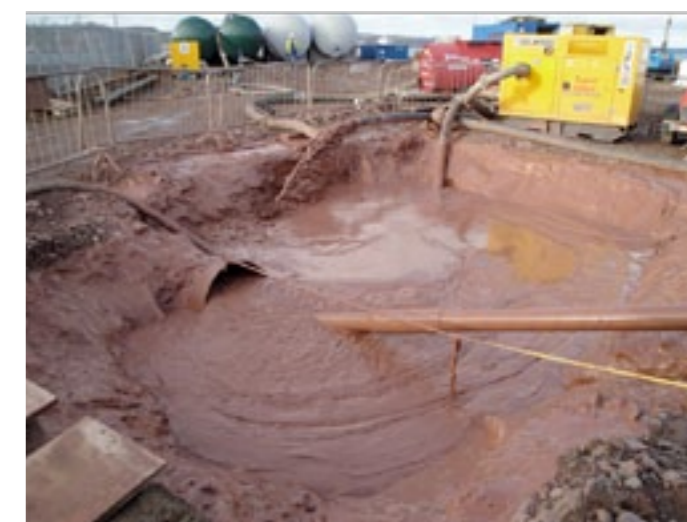
This picture provides an excellent example of shear thinning drilling fluids in action.
