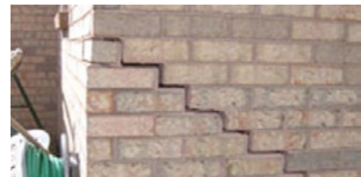
Foundation failures can often be attributed to moisture change in the founding soils
