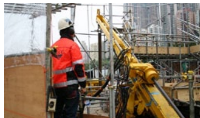
Figure 3: Directional drilling/surveying in a city (Hong Kong) environment (photo courtesy of Devico).
