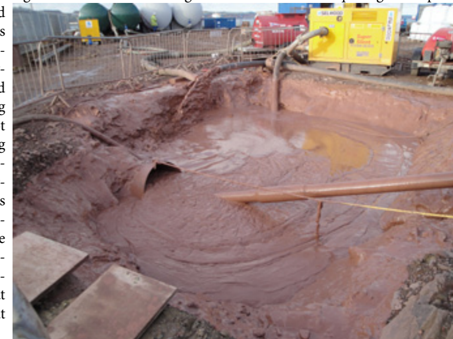
Ultra-Bore® bentonite drilling fluid in use showing exceptional high shear rheology for optimum hole cleaning whilst shearing back down for effective processing on surface.
