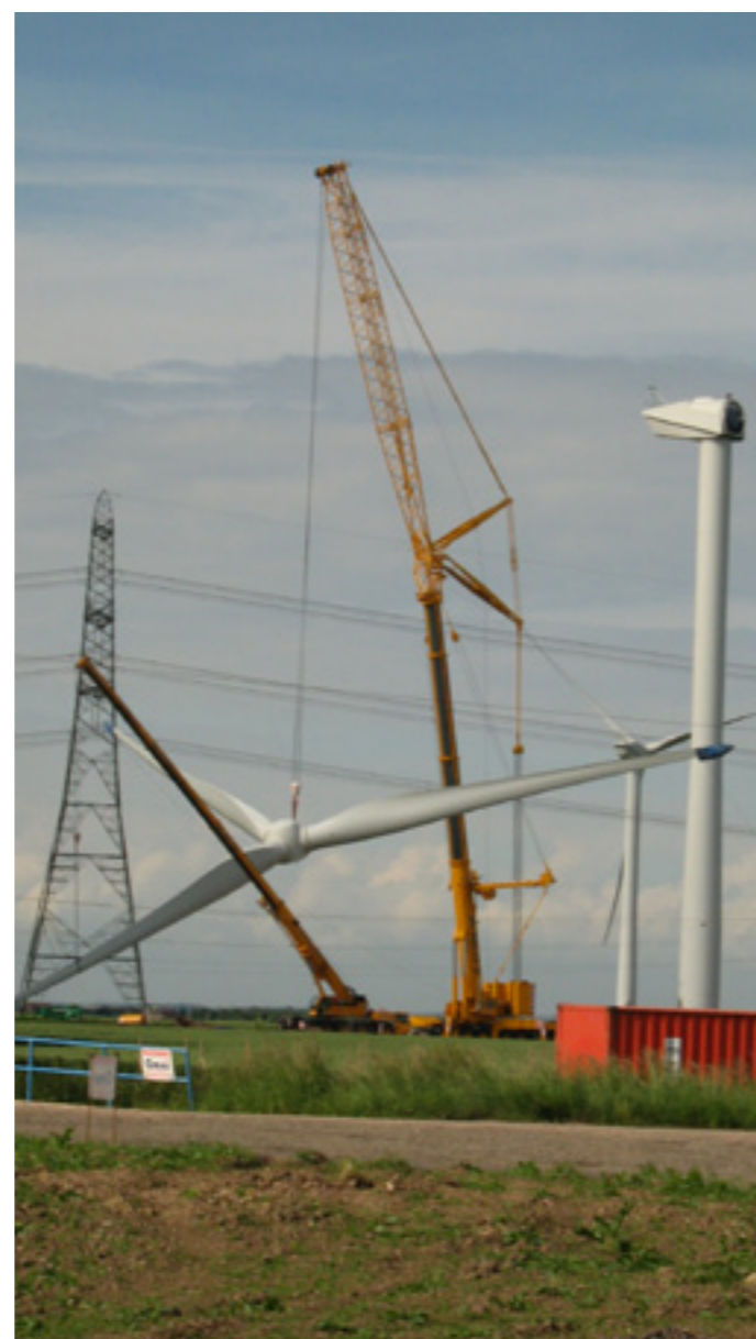
Lifting wind turbine blades into place.
