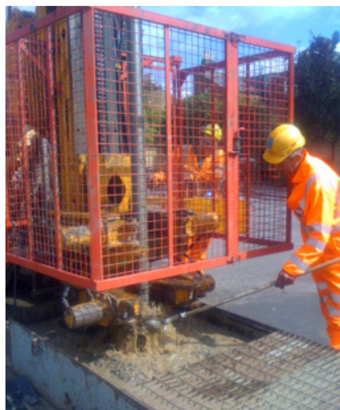
Pure-Bore® drilling fluid effectively stabilising and removing London clay and Lambeth Group cuttings from a geothermal borehole.
