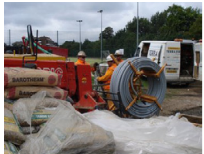
Manual handling has always been an issue on geotechnical sites.
